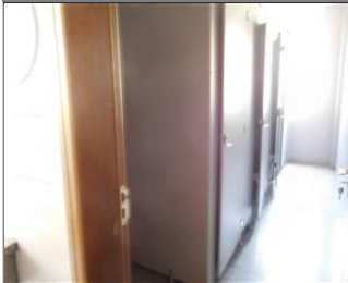
Photo of the sanitary facilities Toilet.JPG
